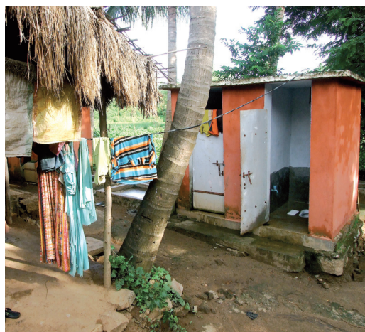
Gram Vikas constructed latrines
