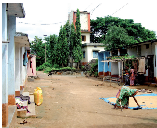
At the back of this Adivasi village can be seen the community water tower constructed by Gram Vikas
